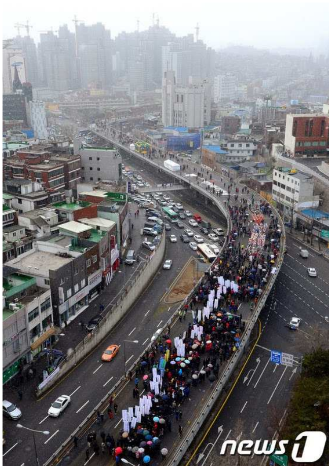
Ahyeon Overpass – NEWS 1
